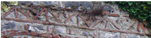
Fig. 57. Castle of Arta. Sections of masonry in 'Alichnotissa' and drawing of detail.
